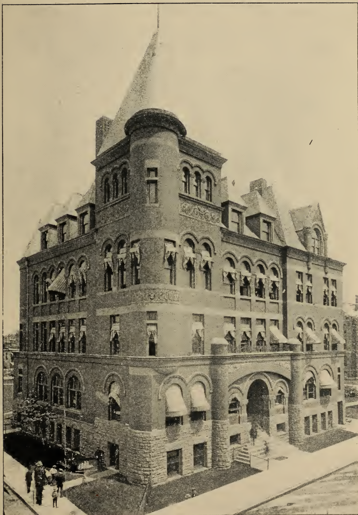
MUNICIPAL COURT BUILDING, Cor. Clinton and Raynor Sts.
